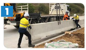
Plan where you want the barriers to be positioned and position close to their final position using a specialist equipment (such as a telehandler).
