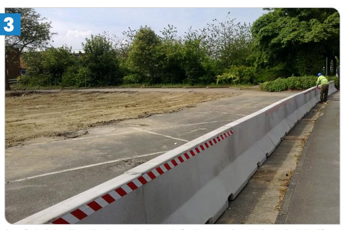
Fix your first barrier in position and butt the second barrier up to the first. The Jersey barriers are designed to interlock and fit together to form a tight join.
