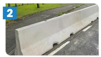
Use forklift truck to position the barriers in the correct place. The distance between the forklift holes on each barrier is 600mm. Each forklift slot 180mm.
